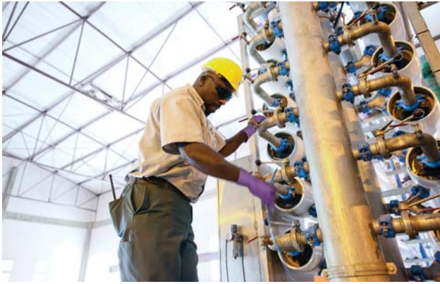
Windhoek has been reclaiming potable water from municipal wastewater for over 50 years. The newest plant features multi-barrier technology (ozone treatment, ultra-membrane filtration and residual chlorination) to eliminate pollutants and contaminants.
