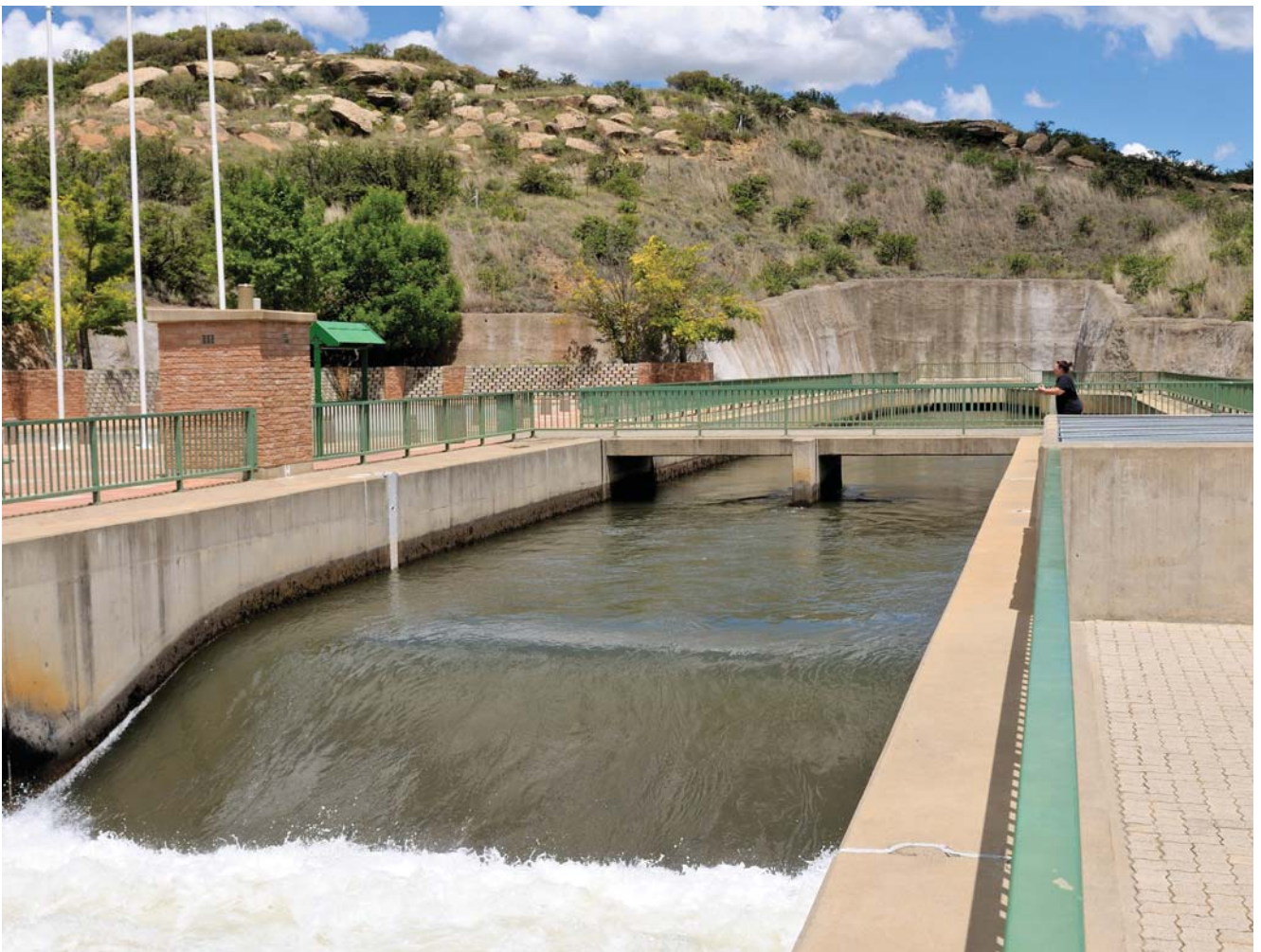
Water enters South Africa from the Lesotho Highlands Water Project. Phase will increase supply from the system by around 15%.
