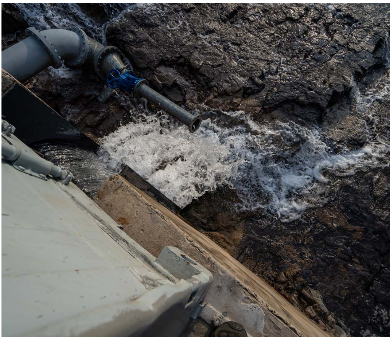
The release from the turbine room is equal to the flow at the intake structure, namely 150 l/s and thus not a consumptive use.
