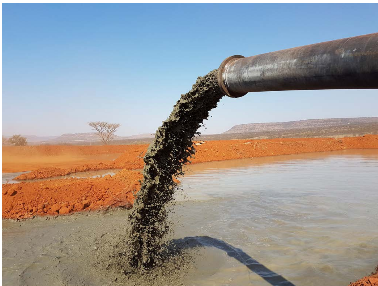
Sediment removal at Oliphantskop dam
