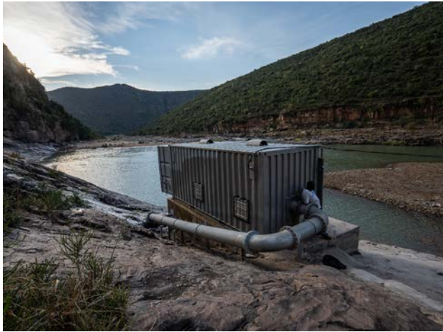
The plant is located inside a retrofitted shipping container and provides enough electricity for approximately 50 rural households.
