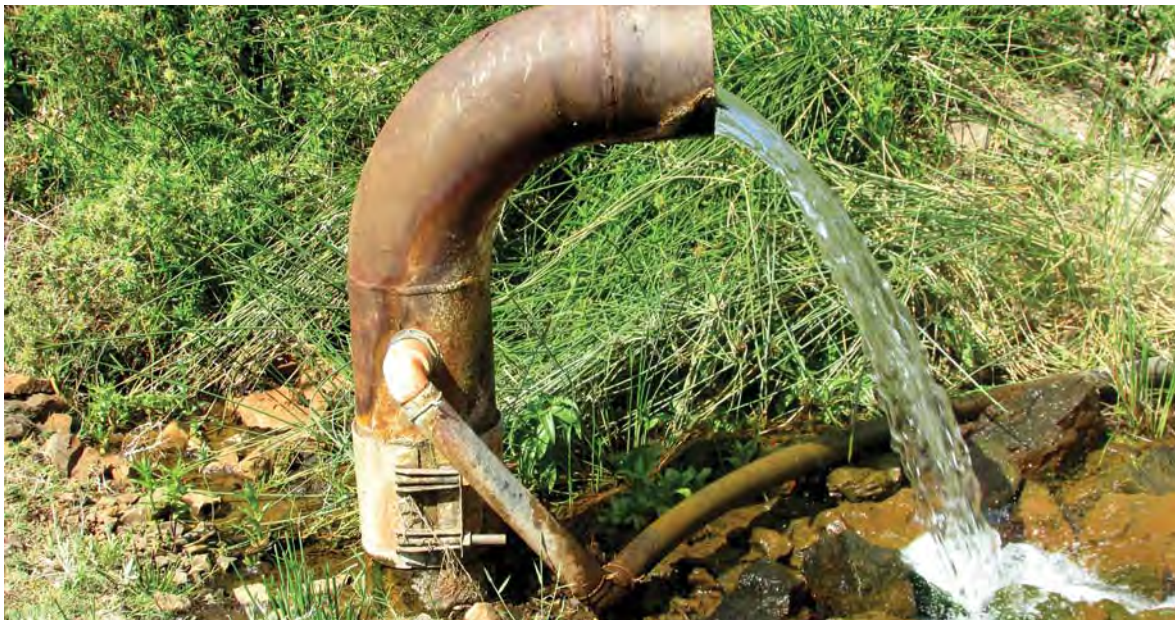
Water spouting from a borehole. If the aquifer is under pressure, groundwater will come to the surface without being pumped.
