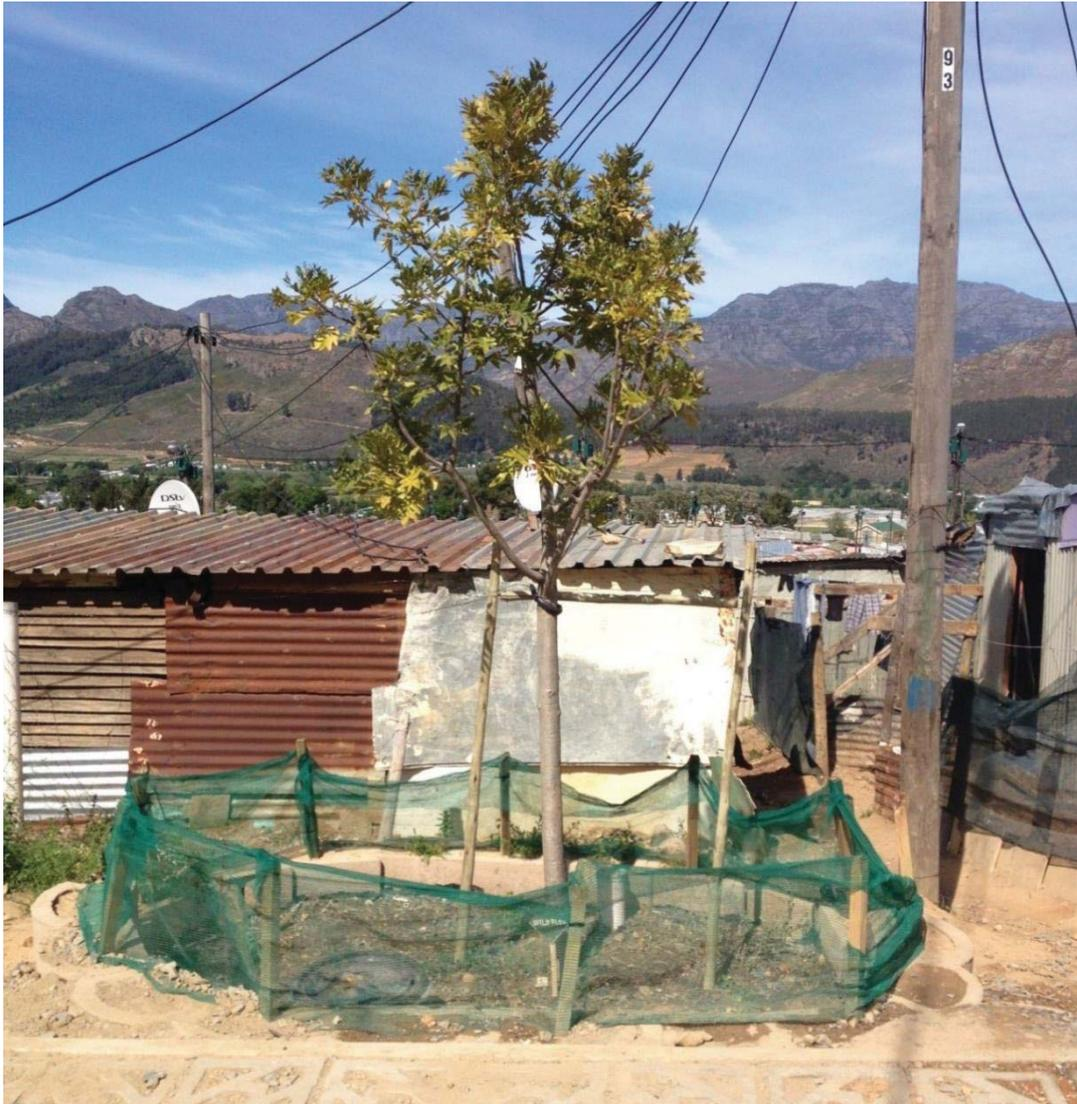
**Figure 3.8** Tree pit for the treatment of greywater in Langrug informal settlement, Franschhoek
