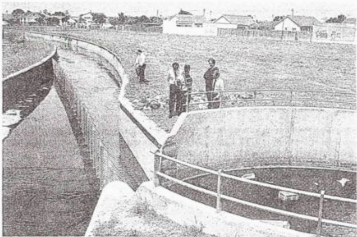
Figure 4-1 : View of the Vygekraal Canal "Enviroscreen"
