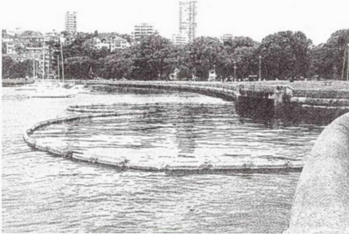
Figure 7-1 : View of a typical floating boom (Rushcutters Bay)
