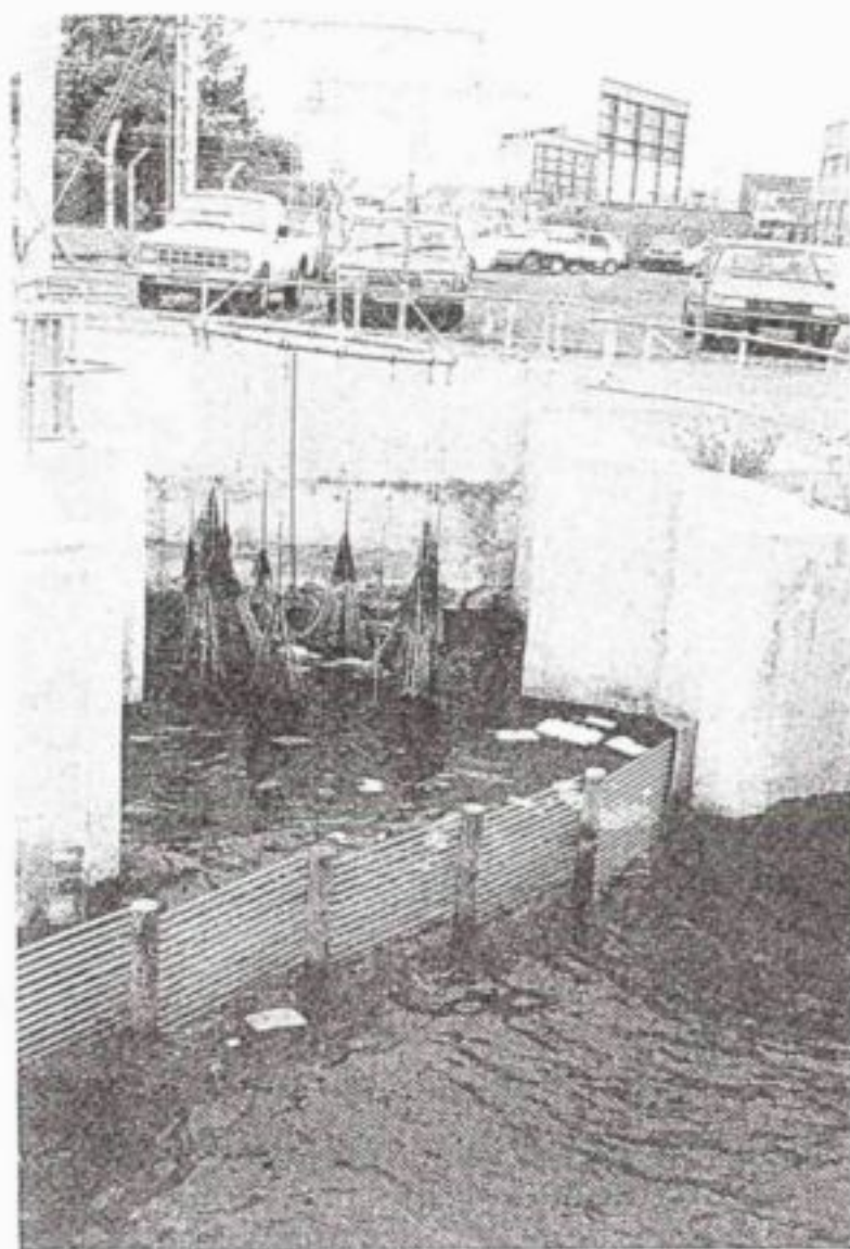
Figure 4-2 : View of the Mullet Stream "Enviroscreen" showing the net and lifting ring provided to remove the litter from the sump
