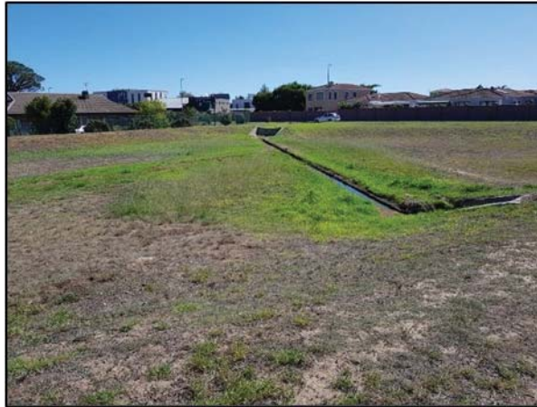
Figure 2-5: Detention Pond in residential areas, Somerset West (2021)
