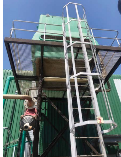
Figure 10-9: Photo Image of a Cooling Tower at Afro Fishing that assists in Retort Cooling after Cooking
