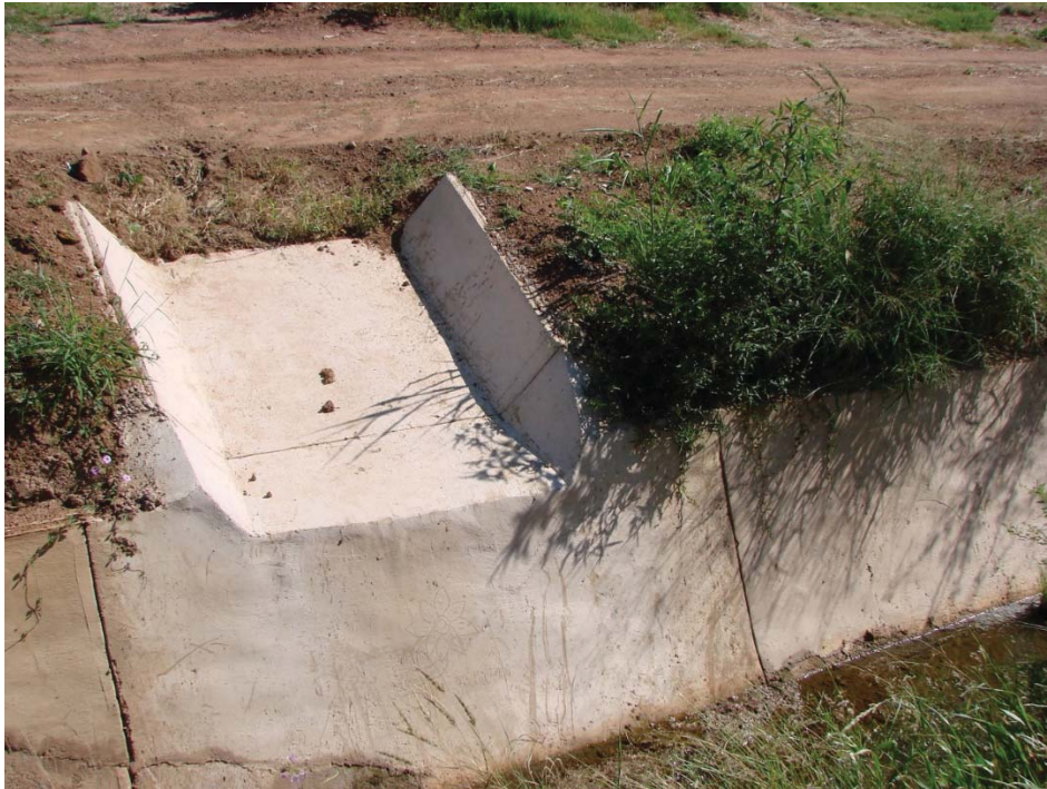
Figure 108: Storm water inlet for water entering drainage canal DG4
