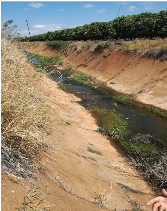
Figure A14: Drainage canal DJ5
