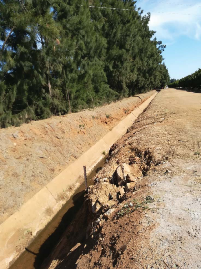
Figure A15: Drainage canal DJ13
