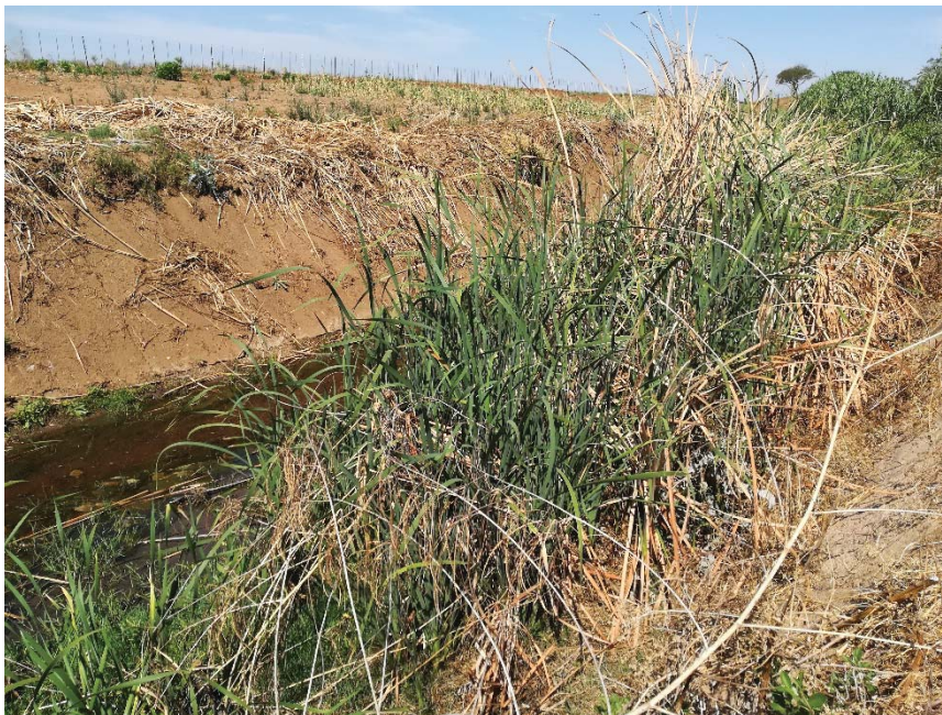
Figure A18: Drainage canal DJ8
