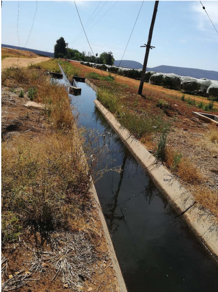
Figure A11: DH5 irrigation canal
