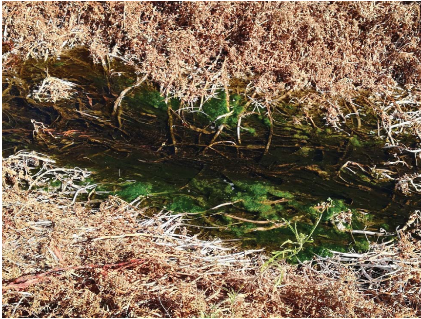
Figure A17: Drainage canal DF2
