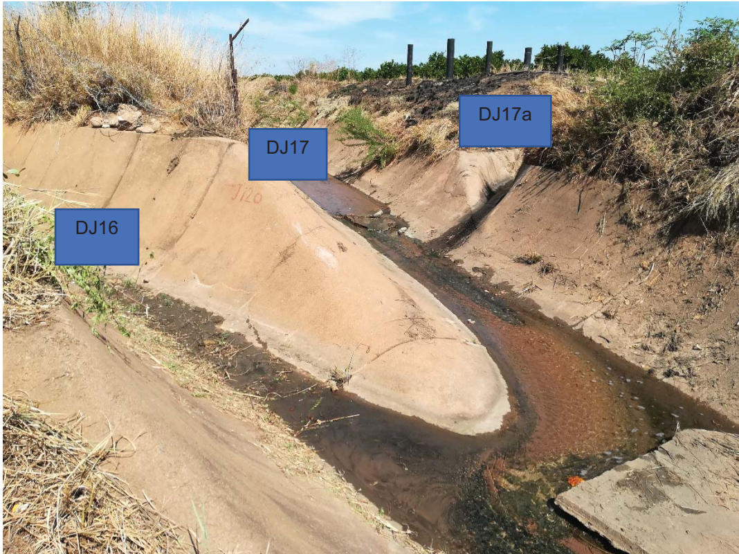
Figure A13: Confluence of drainage canals consisting of DJ16, DJ17 and DJ17a
