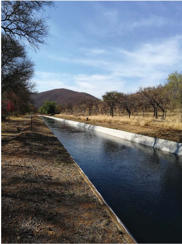
Figure A9: Loskop Nature Reserve irrigation canal
