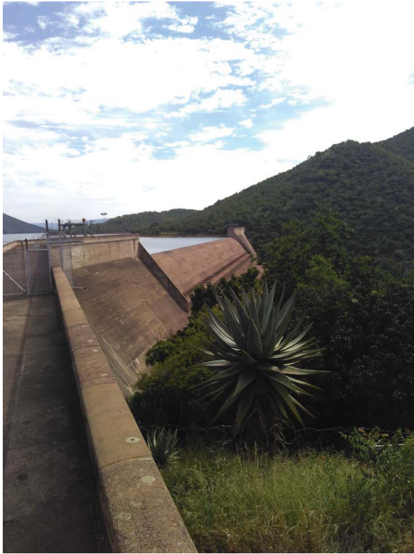
Figure A1: Loskop Dam wall
