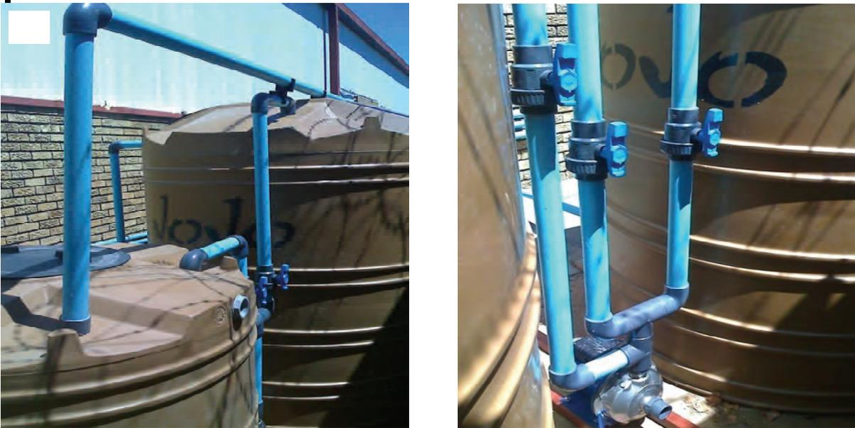
**Figure 4.9** (A) Reticulation for 10,000 L equalization tank. (B) Recycle configuration between anaerobic and anoxic tanks.
