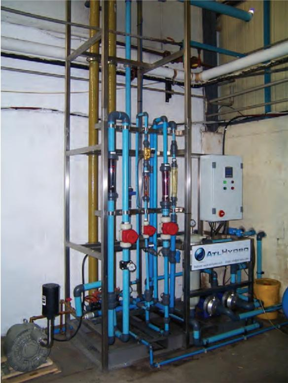
**Figure 4.12:** MBR pilot plant ultrafiltration unit indicating Norit X-Flow Airlift™ pilot modules relative to pumps and pre-filter.
