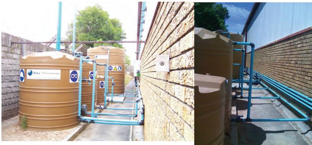
**Figure 4.8:** (A) EPBR and pre-denitrification MBR configuration: 1. Equalisation; 2. anaerobic; 3. anoxic; 4. aerobic. (B) Reticulation to the sump and MBR UF unit; sump distance 50 m; MBR unit distance 36 m
