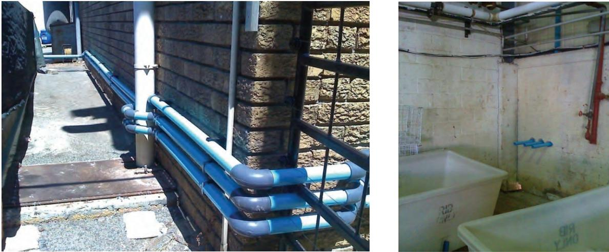
**Figure 4.11:** (A) Reticulation entry point into sump and municipal drain (overflow design); (B) aerobic tank reticulation entry point into dye house – the MBR unit was connected to these pipes.
