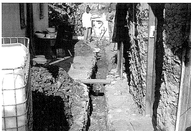
Pilot initiative to implement shallow sewerage technology in Durban. (Proj No 1146).
