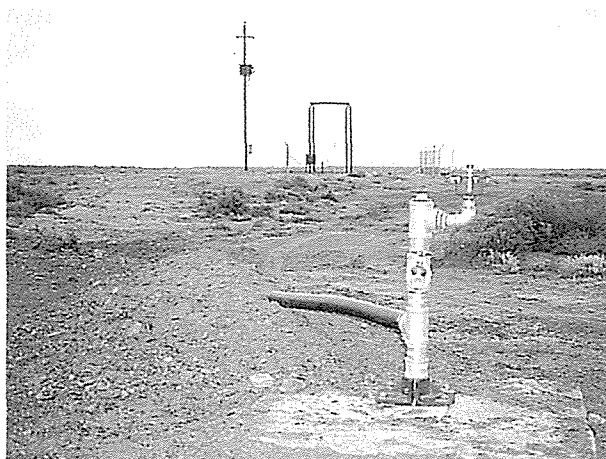
One of the injection boreholes, with the abstraction borehole in the background (near Calvinia, Karoo).
