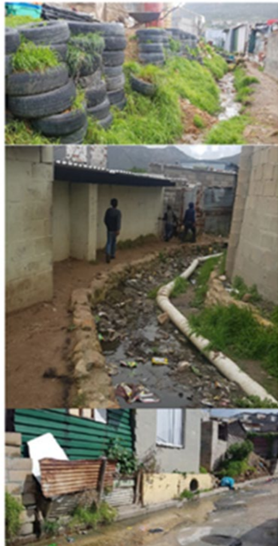
Figure 59: Drainage systems in Hangberg (Smith, 2020)
