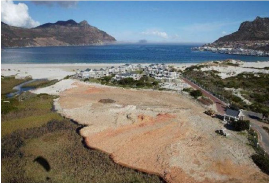
Figure 39: An aerial view showing the infilling of the Disa [Hout Bay] River floodplain as part of the Beach Club housing development. (Photo by Anthony Allen, CA, 2011)
