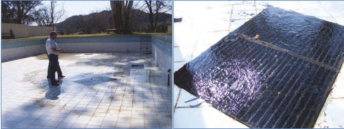
Photos 11 & 12. Cradock spa swimming pool in August 2013 (after being drained for cleaning), with metal grids protecting the bubbling springflow from below (photo courtesy S Mullineux, DWA, Cradock).
