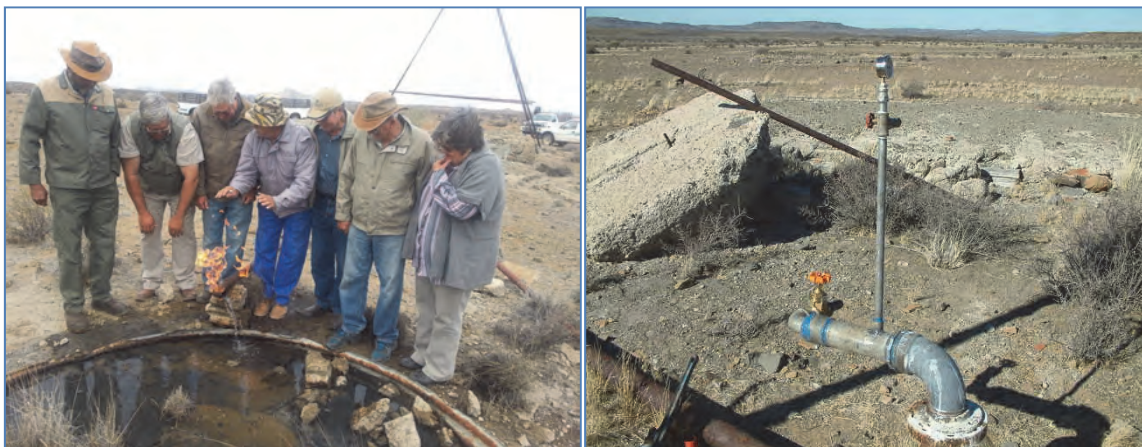
Photos 19 & 20. Burning gas at the outlet pipe; and the new valve and pressure gauge installed by the IGS, University of the Free State
