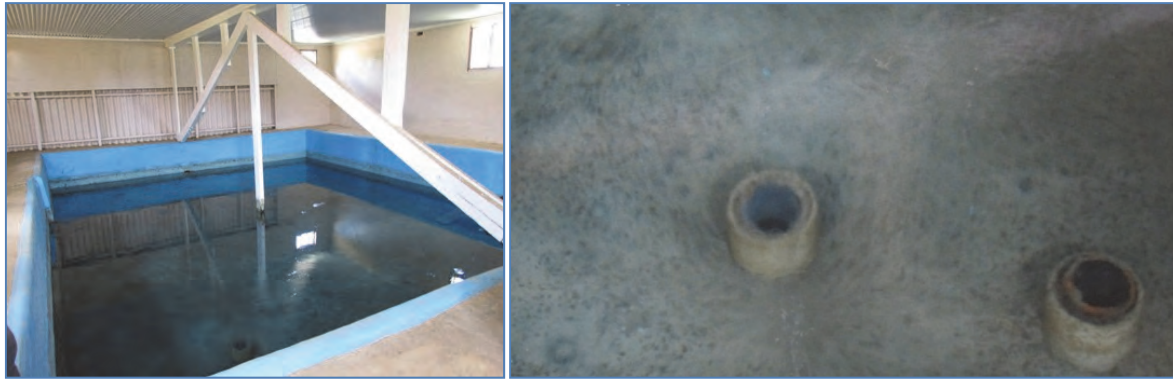
Figure 1: Florisbad spring pool and ~10cm diameter pipes at the base of the pool from which the spring flow discharges into the pool.
