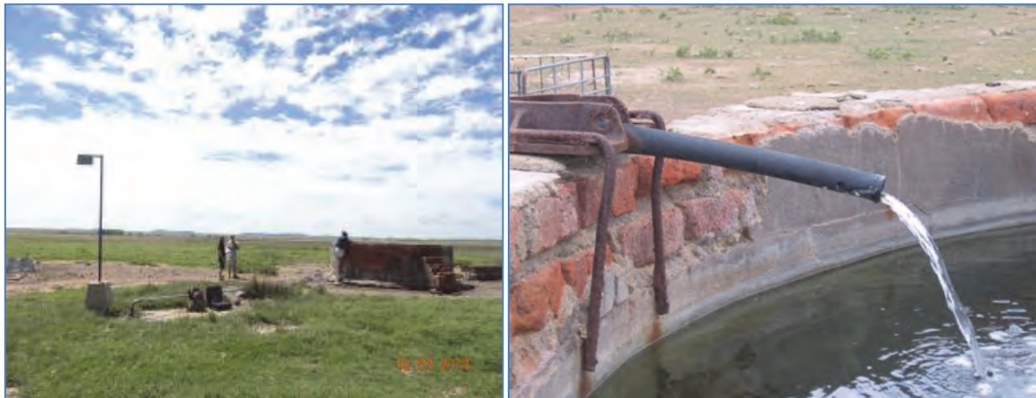
Photos 3 & 4. The artesian borehole (located next to the beacon), and its discharge into the nearby reservoir.
