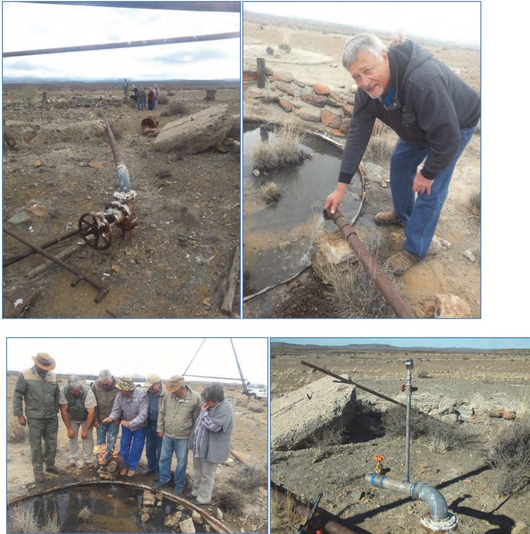
Figure 27: SA1/66 being opened for the first time in about 50 years showing water and inflammable gas discharging.
