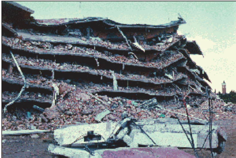
Figure 3: The 1976 Welkom seismic event in which a block of flats, six storeys high, collapsed. (Photographer unknown)
