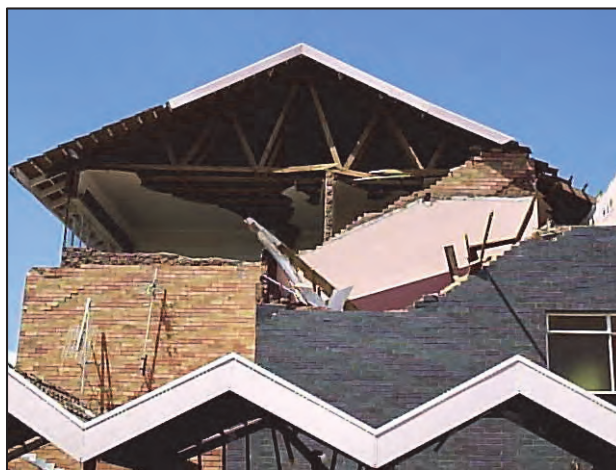
Figure 1: Effect of the 2005 Stilfontein seismic event of M_L 5.3 on the A-block of the Bal-Eaton flats. (Photo courtesy of Ian Saunders, Council for Geoscience, Pretoria)
