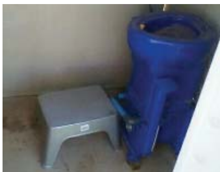
Positioning of the water dispenser, toilet sink and urinal
