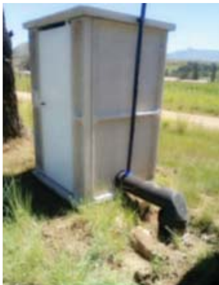
The superstructure with air vent.
