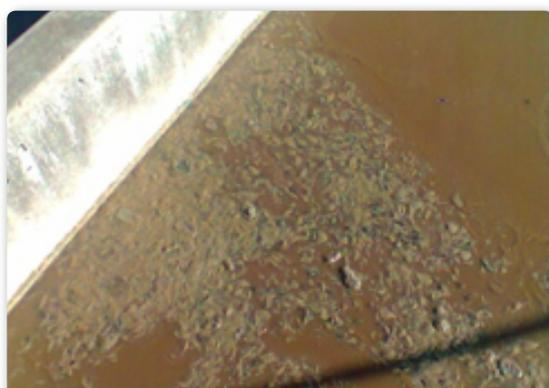
*Figure 3: Feathers collected in one of the corners of the activated sludge reactors in Hartbeesfontein*
