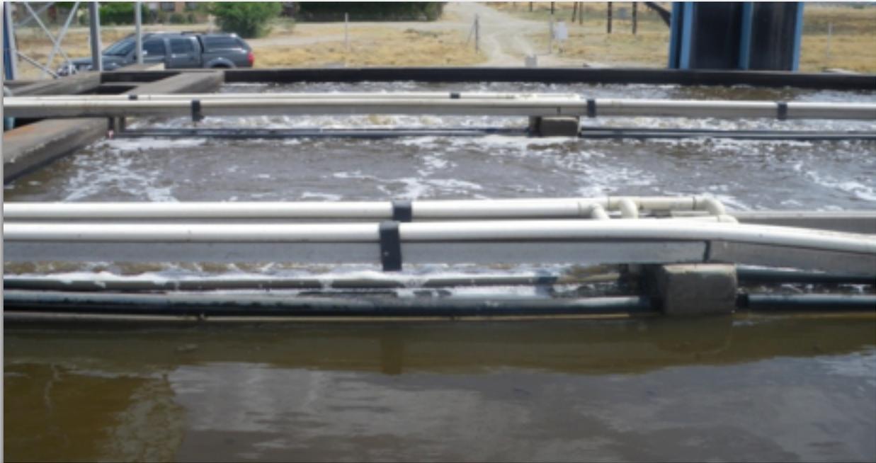
**Tokologo** – Close circuit wastewater treatment tank divide into three compartments of equal volume
