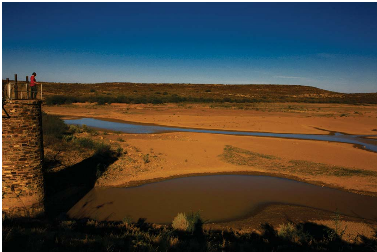
The Vanwyksvlei Dam is more often than not dry.
