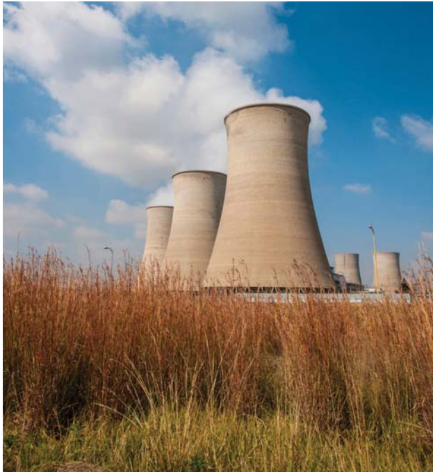
The cooling towers of the Grootvlei power station. While the old, recommissioned Eskom power stations are helping to meet the demand for electricity they are not as water efficient.
