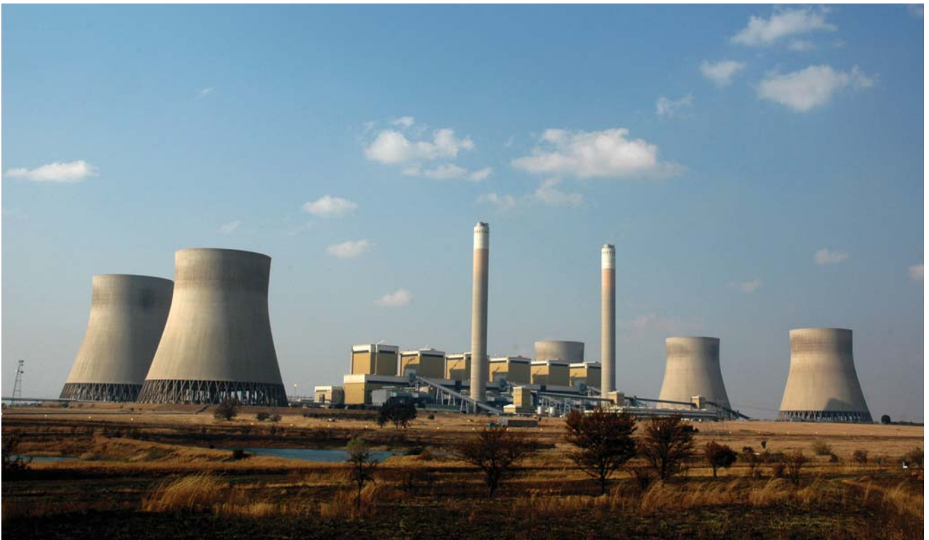
Kendal power station, outside Witbank in Mpumalanga is one of the largest dry cooled power stations in the world. The water consumption of South Africa's dry cooled power plants is among the best in the world.
