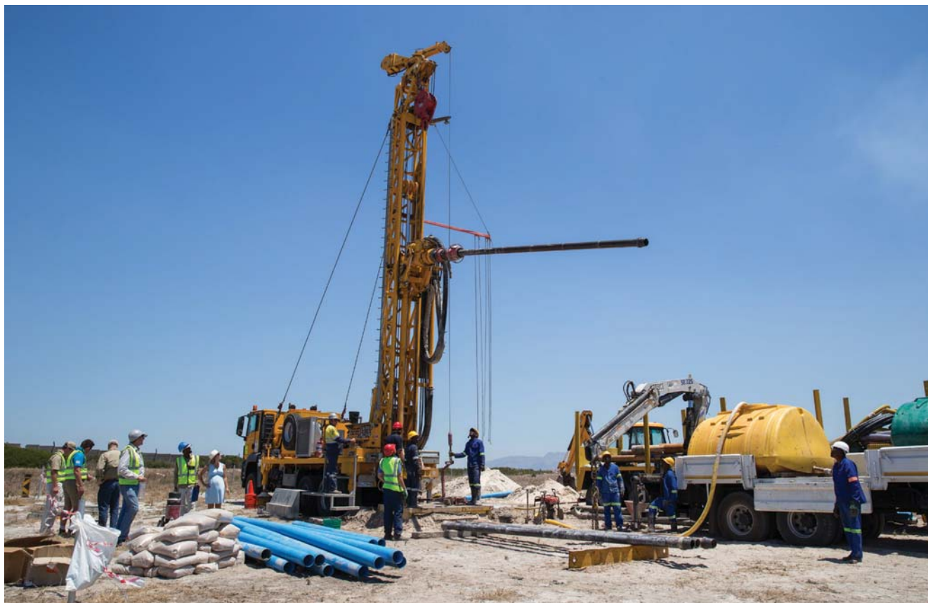
Drilling for groundwater during the height of the Cape Town drought.
