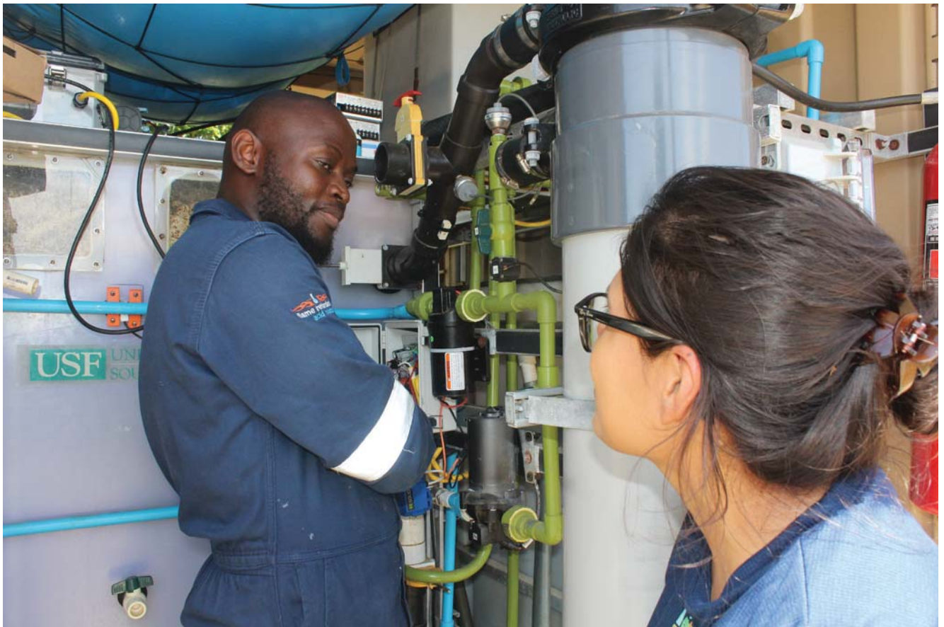
PRG engineer, Lindelani Xaba, and University of South Florida postdoctoral scholar, Dr Cynthia Castro, discuss the operation of a prototype water-saving system at a community toilet block in the Durban North area. The system, designed by the University of South Florida, saves water by passing wastewater through an anaerobic digester and advanced membrane filters. The recycled water is used to flush toilets
