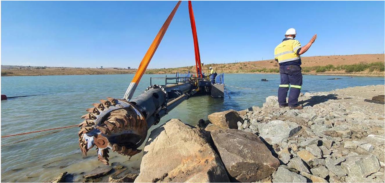
The business end of a cutter suction dredger at Mvunyane dam.
