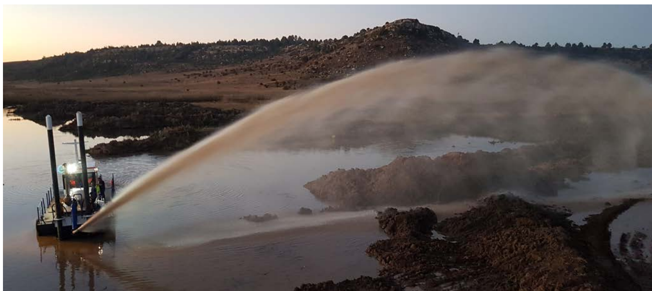
Dredging is one option available to physically remove decades of silt build-up from South Africa's dams.
