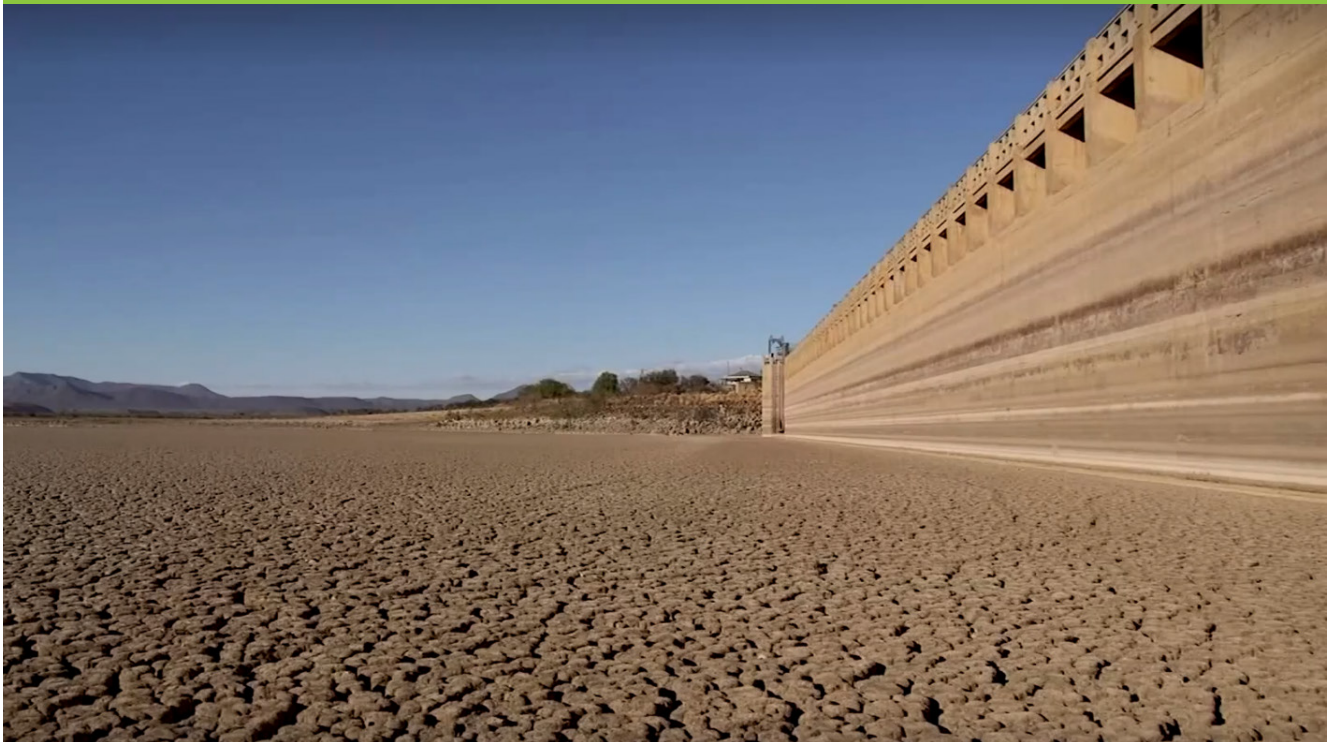
The Nqweba Dam was built in 1925 to provide irrigation. But over the last 96 years the dam has lost more than 40% of its water storage capacity due to siltation and currently has very low water levels.
