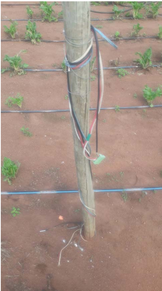
Chameleon sensor at Rooiwal, abandoned and disconnected.
