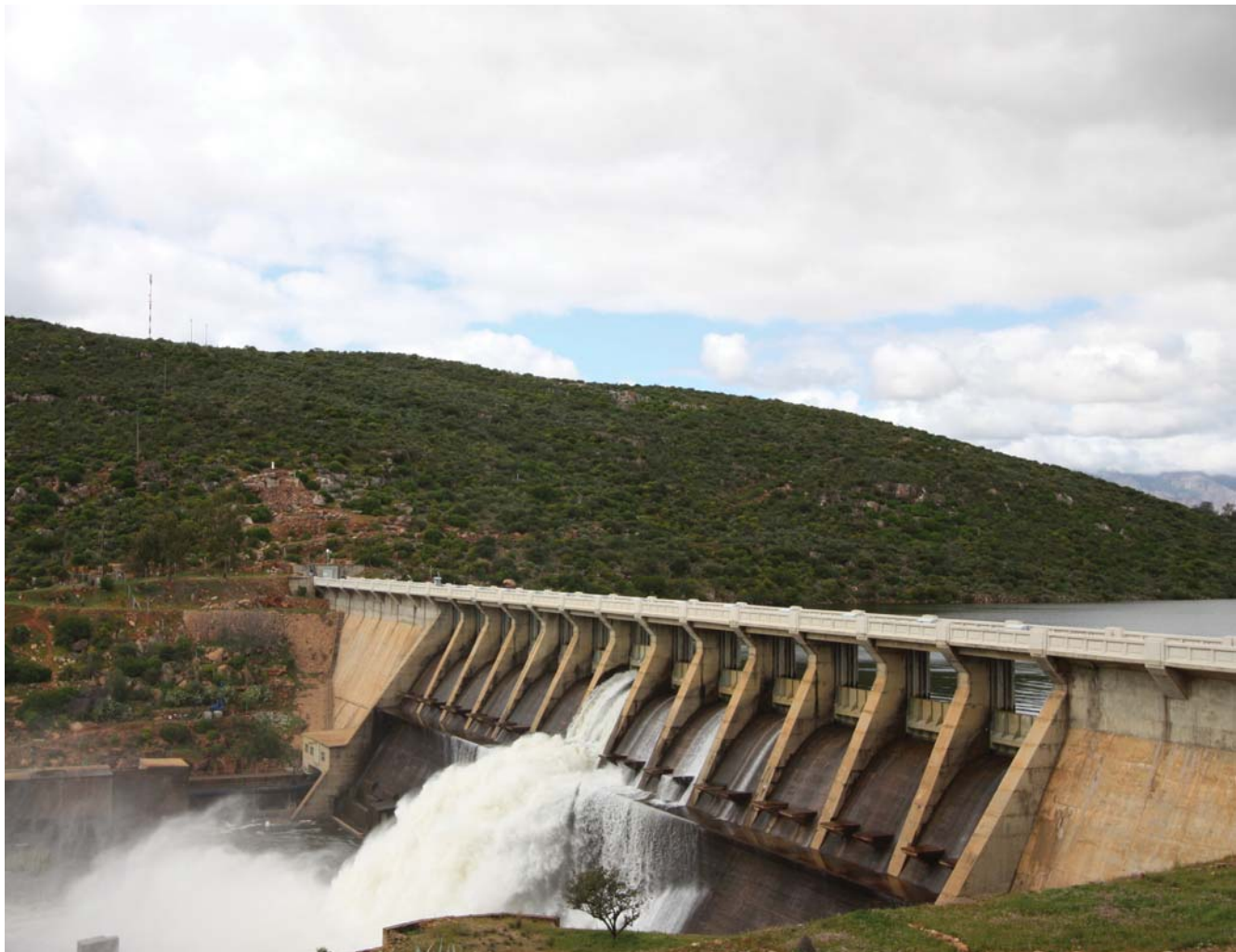
Clanwilliam Dam has a current capacity of close to 122 million m 3 .
