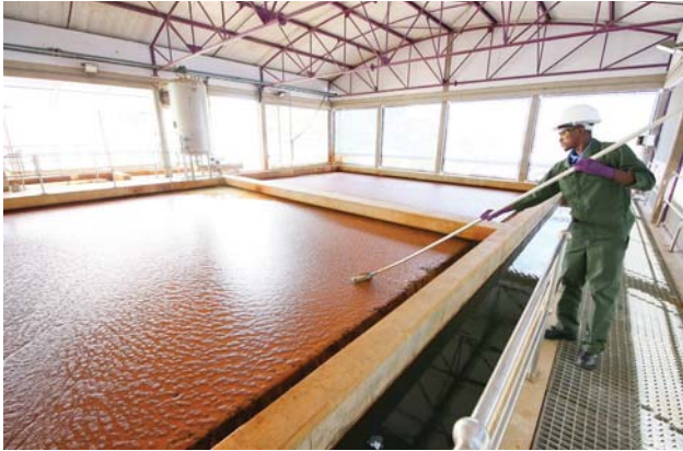
Above and top: Windhoek has been reclaiming potable water from municipal wastewater for over 50 years. The newest plant features multi-barrier technology (ozone treatment, ultra-membrane filtration and residual chlorination) to eliminate pollutants and contaminants.
