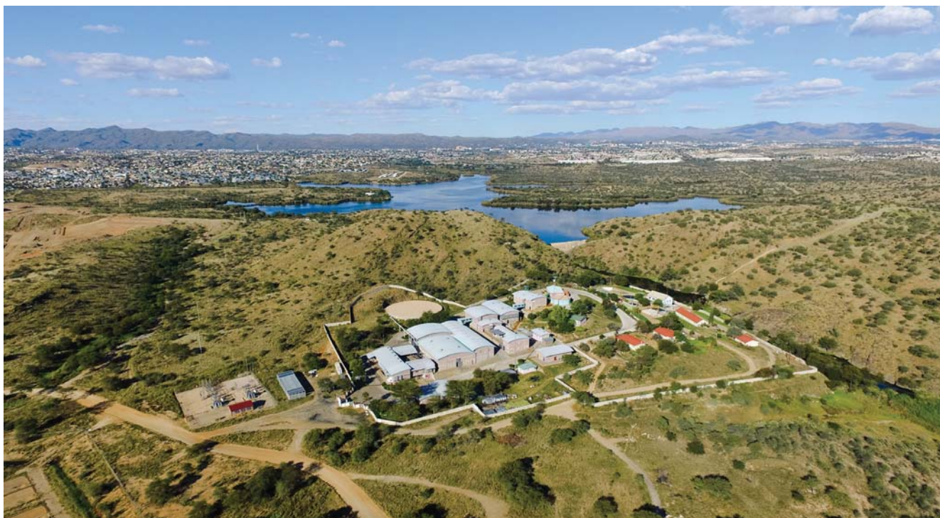
An aerial view of the Windhoek water reclamation plant and Goreangab dam. The Namibian facility, the first plant of its kind in the world, was established in 1968.
