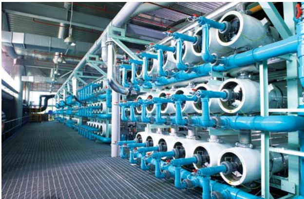
Singapore has been reclaiming high quality water from municipal wastewater for nearly two decades. The biggest users are semiconductor wafer fabrication plants, which require water quality even more stringent than potable water.
