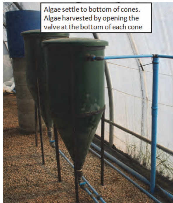
Figure 2.7 The algal setting cones in which algae were separated from the effluent drawn from the high rate algal ponding (HRAP) system before the treated water was moved to either the constructed wetland (CW), hydroponic or aquaculture system (Photo: Rory Scheepers).
