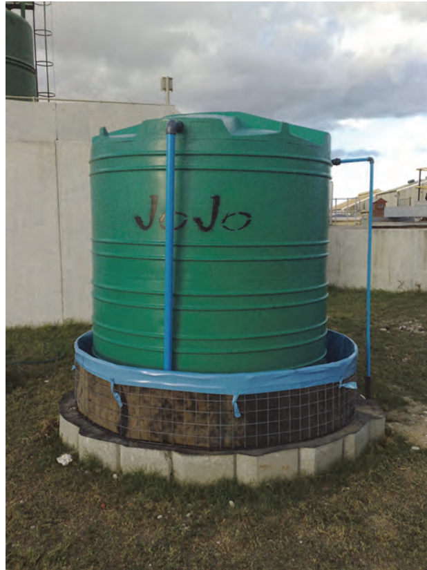
Figure 2.2 The 5000 L holding tank in which post-anaerobic digester (post-AD) effluent was held prior to entering the primary facultative pond (PFP) (Photo: Rory Scheepers).
