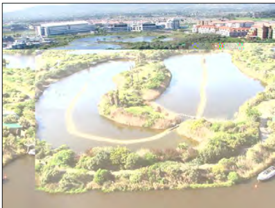
Figure 5.4: Constructed wetland, Century City, Cape Town
