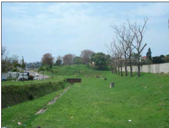
Figure 5.1: Large roadside detention pond, Hillcrest
