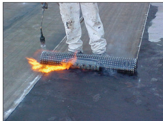
Figure 3.2: Waterproofing a roof in preparation for the construction of a green roof
