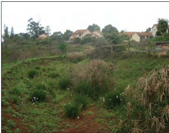
Figure 4.3: Swale combined with bioretention areas, Hawaan Estate, Umhlanga
