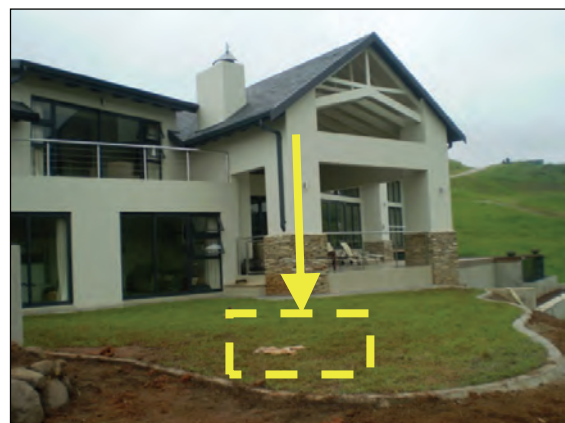
Figure 3.5: Groundwater recharge of runoff from a single residential dwelling, Cotswold Downs Estate, Hillcrest
