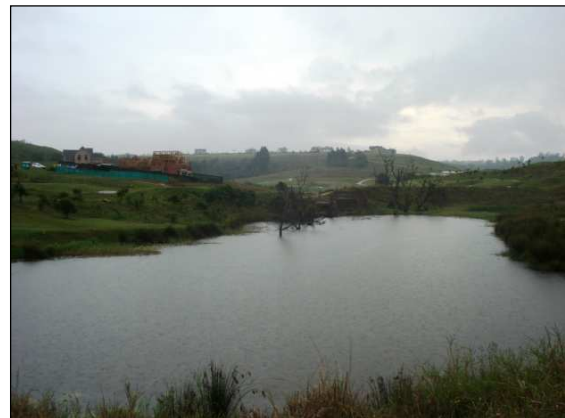
Figure 5.3: Large retention pond, Cotswold Downs Golf Estate, Hillcrest
