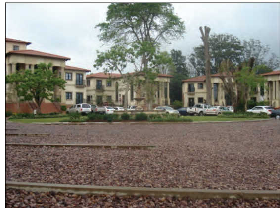
Figure 3.8: Gravel pavement system, Bishops Court Office Park, Hillcrest
