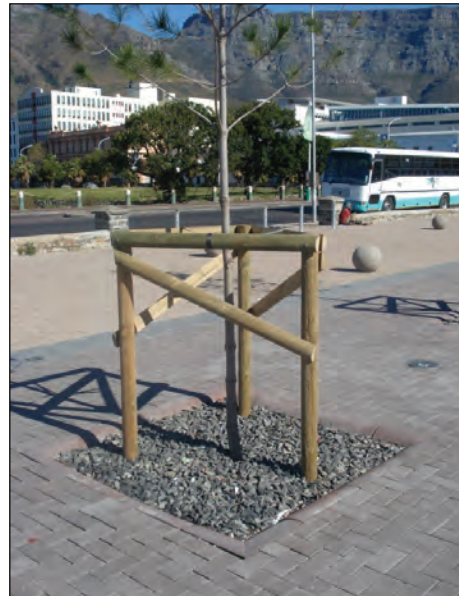
Figure 4.6: Bio-retention rut filled with a coarse aggregate and planted with a tree, Grand Parade, Cape Town
