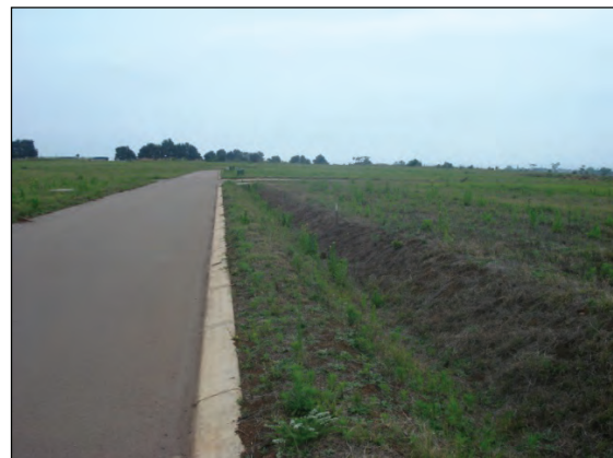
Figure 4.2: Roadside swale, Cotswold Downs Golf Estate, Hillcrest
