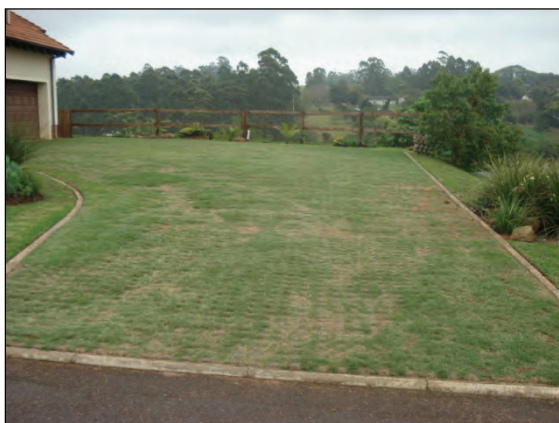
Figure 3.9: Modular pavement system planted with grass, Clifton Hill Estate, Hillcrest
