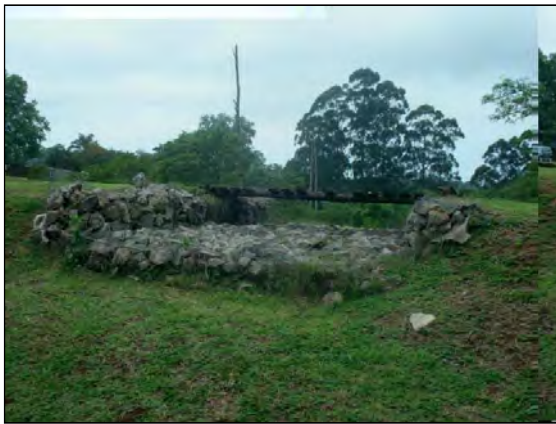
Figure 5.2: Detention pond emergency overflow structure, New Heritage Market, Hillcrest
