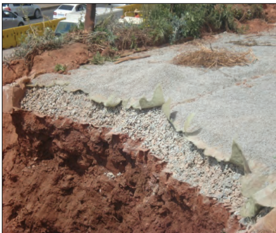
Figure 3.7: Section through the base layers that will support permeable concrete block pavers
