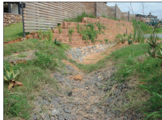
Figure 4.4: Gabion-lined dry swale, Hawaan Estate, Umhlanga
