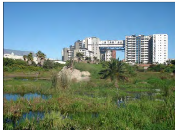
Figure 5.5: The macrophyte zone in a constructed wetland, Century City, Cape Town
