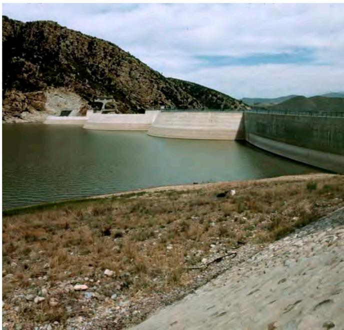
**Left:** *Stompdrift Dam has a full storage capacity of some 49,6 million m<sup>3</sup>.*
