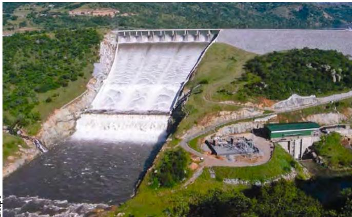
Maguga Dam's labyrinth spillway has one of the highest capacities of its type in the world.
