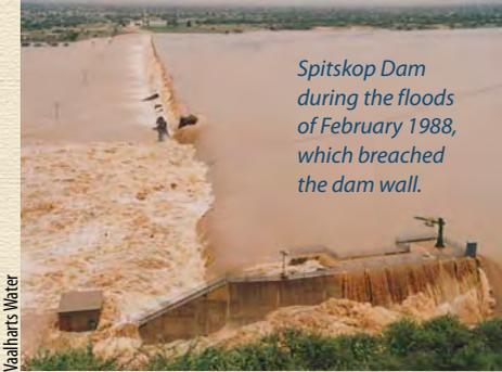
*Spitskop Dam during the floods of February 1988, which breached the dam wall.*
