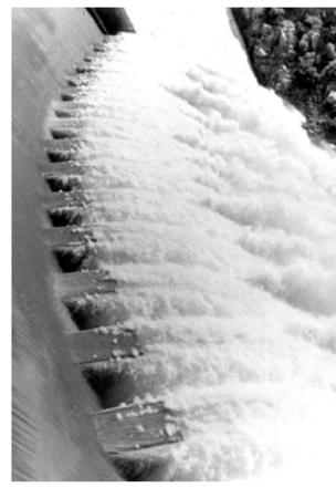
**Top left:** Blyderivierspoort Dam is a concrete gravity arch dam. It was one of the first dams in the country where computers were used in the design calculations.
