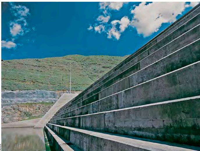
**Bottom right:** Commissioned in October 2001 the Matsoku Weir and tunnel increases the supply of the Katse reservoir by transferred up to 55 m<sup>3</sup>/s into the dam during high flow conditions. The weir's downstream face features a series of large steps, designed to dissipate the energy of water overflowing the weir.
