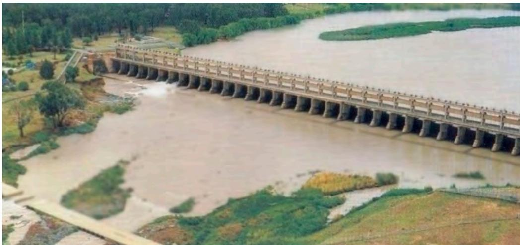
*Vaal Barrage from the air. Here the 36 sluice gates can clearly be seen. Each gate measures 7,5 m by 9,6 m and weighs about 26 tons.*
