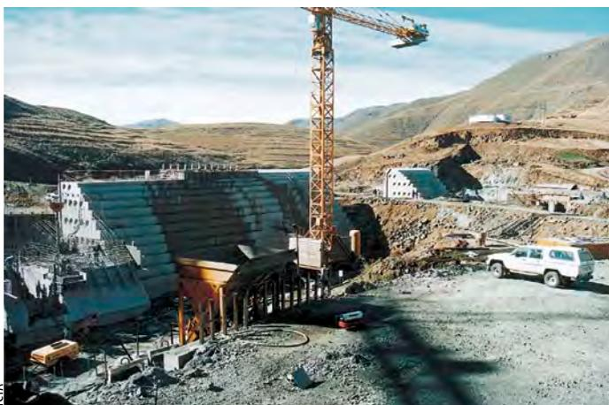
**Bottom left:** Matsoku weir during construction. The 15 m-high weir is situated on a bend in the Matsoku River about 12 km north of Katse Dam.
