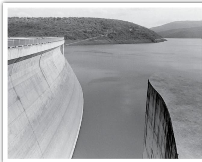
**Below:** Pongolapoort Dam as seen from the air. The dam has gross capacity of 2 500 million m<sup>3</sup>- twice the mean annual runoff of the river.
