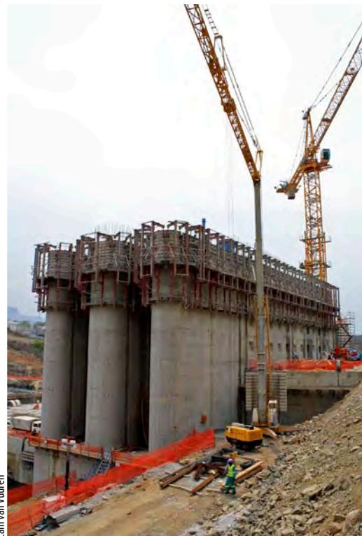
The multi-level outlet structure of De Hoop Dam. The outlet works will have a maximum capacity of 20 m<sup>3</sup>/s – 15 m<sup>3</sup>/s of which is to meet Environmental Reserve requirements.
