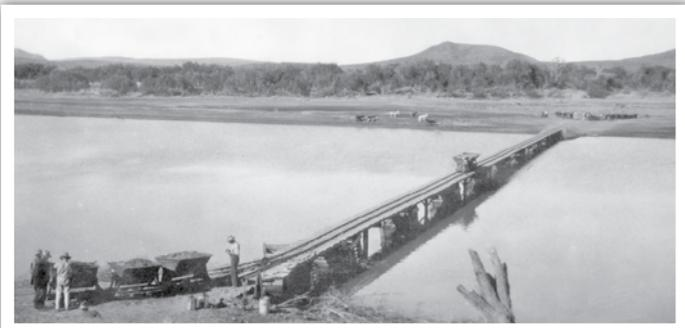
**Top left:** *The temporary bridge over the Orange River providing access to the sand island. Sand was brought to site on cocopans.*
