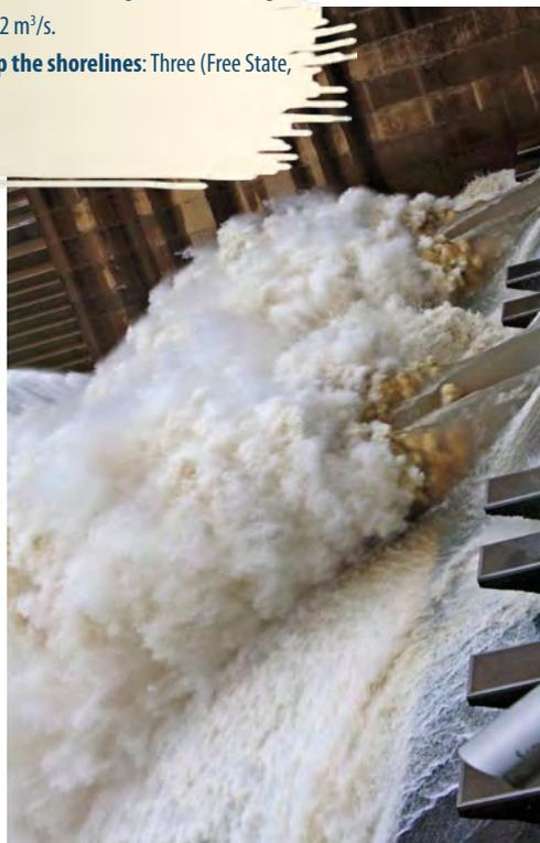
**Above:** The Vaal Dam is a concrete gravity structure with an earthfill section on the right flank. The dam has a current capacity of 2 536 million m<sup>3</sup>.
