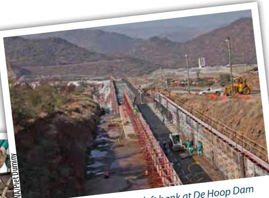
A general view of the upper left bank at De Hoop Dam as it stood in June 2011. Note the specially-designed scaffolding.
