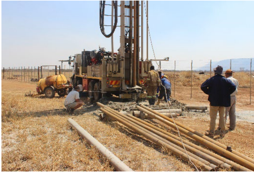
Figure 2: Pumping boreholes in Mamadila
