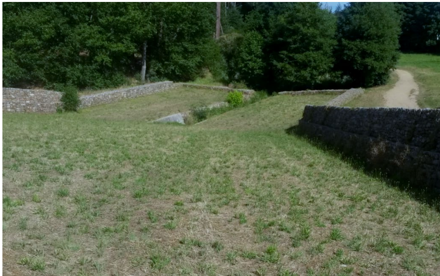
Figure 5.2: Detention ponds along Constantia Alphen green belt (Source: De Chavonnes Vrugt, 2016)
