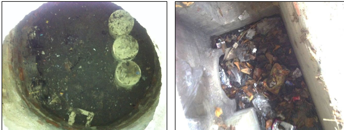
Figure 5.6: Sediment in inlet manhole (left) and debris blocking roadside inlet (right)
