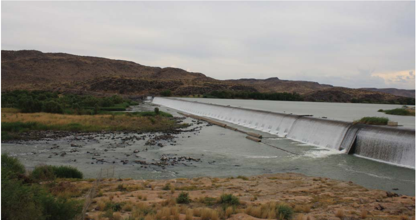
The Buchuberg Dam on the Orange River.
